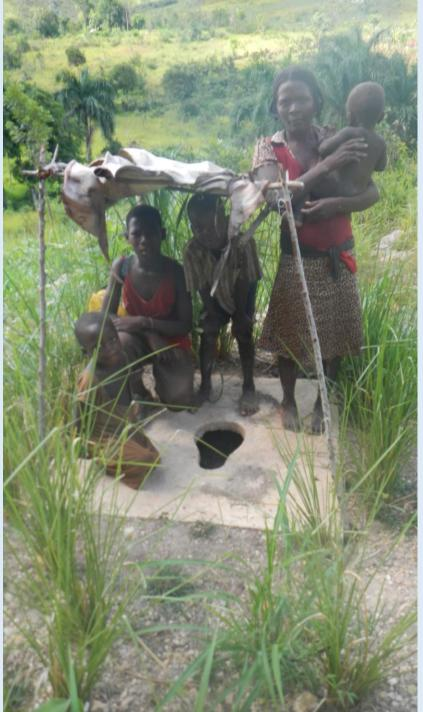
A Vetiver toilet is simply Vetiver grass slips planted around a small concrete slab above the pit. Instead of bricks and mortar the long roots of the grass stabilize the pit and even remove environmental contaminates.
